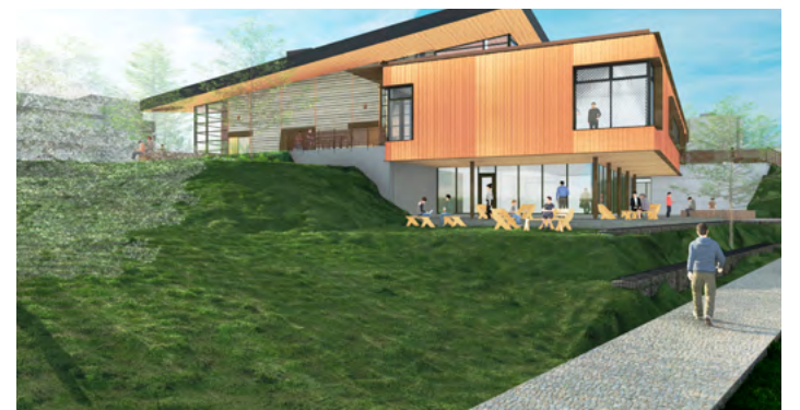
View from south west of multi-generational lounge and outdoor gathering (great hall beyond)
